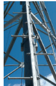
Welded Sections used on sections #13-21
