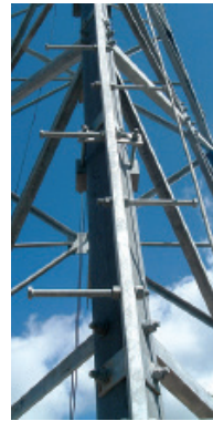
Welded Sections used on sections #13-21
